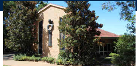
St Brigid's Chapel and Religious Education Centre opened in November 2001, providing flexible learning and sacred spaces for the College
